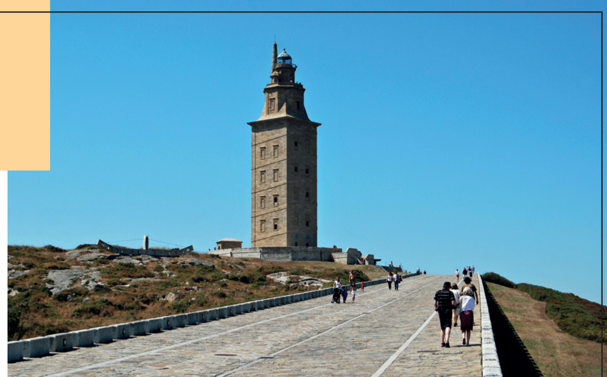
Hercules Tower, A Coruña
