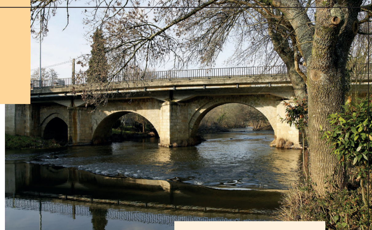
Bridge over the Tambre river, Sigüeiro
