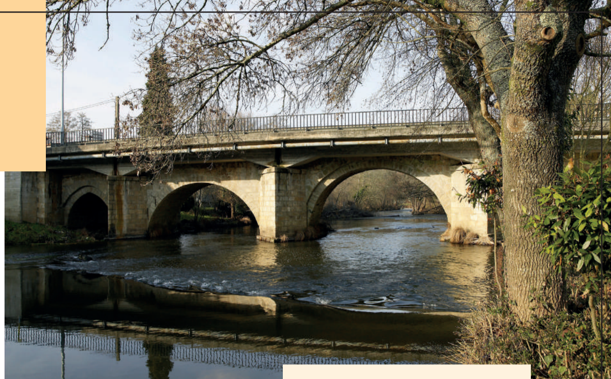
Bridge over the Tambre river, Sigüeiro
