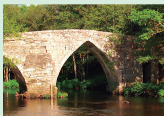
Santo Alberto Bridge, Guitiriz
